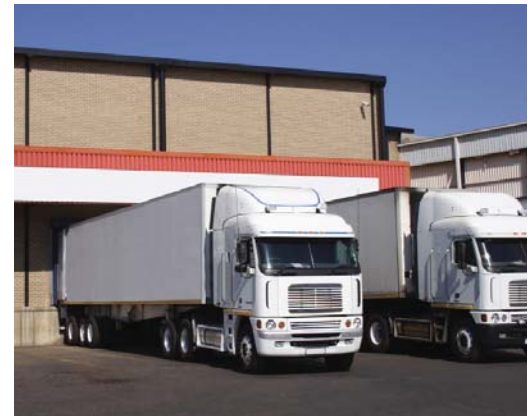
Loading bay of large cold store.
